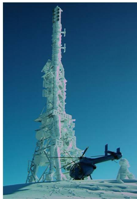
Figure 7-13: A broadcasting tower (continuing to function in ice / snow conditions)
